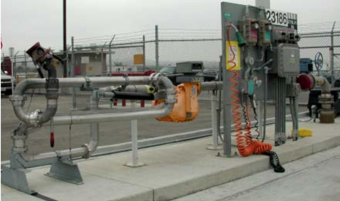
Refueling of tank trucks with bottom loading connection
